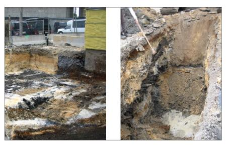
Typical test pits in geo-environmental engineering site soil characterisation. One attribute rules the day: "significant heterogeneity". It is obvious that any single field sample (a grab sample in the TOS parlance) will not be able to represent the entire site. For this job, diligent compliance with the TOS' principle of *composite sampling* is necessary (see part 2).
